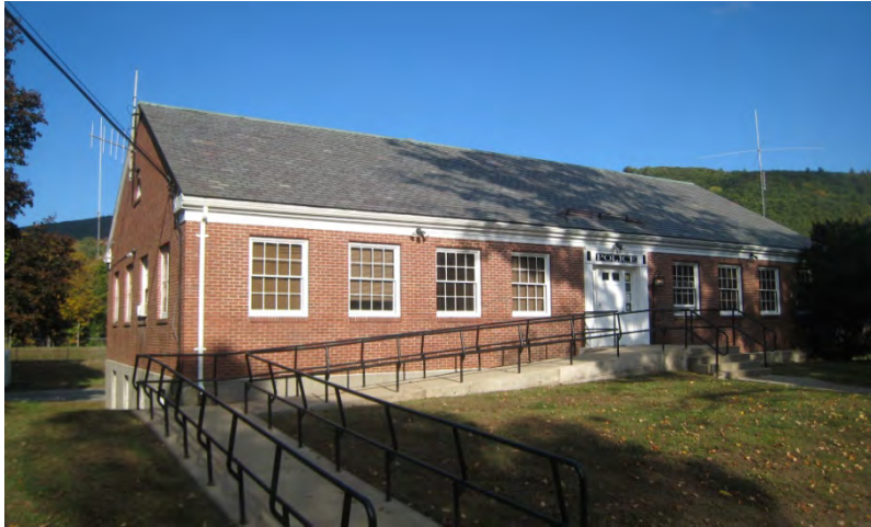
View from Conway Street
