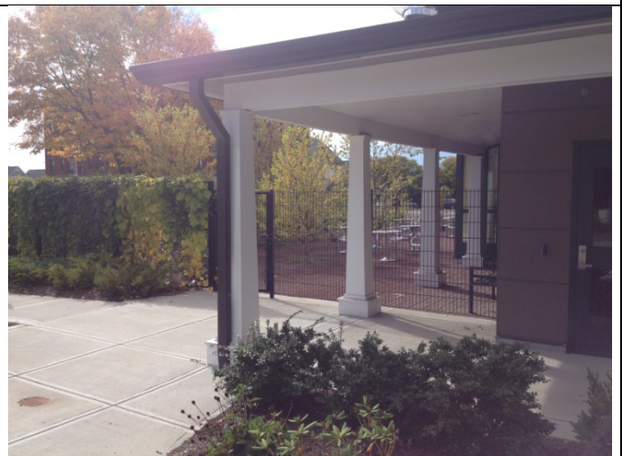
10. Covered porch at main entry
