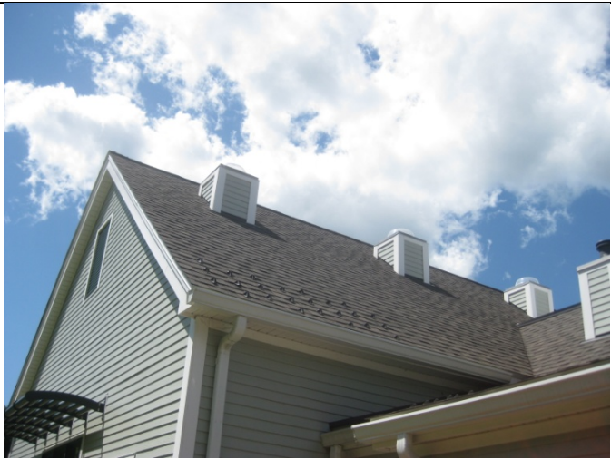
11. Light tubes at roof, provide natural light into building
