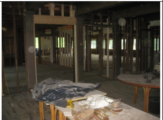
10. Partially renovated first floor
