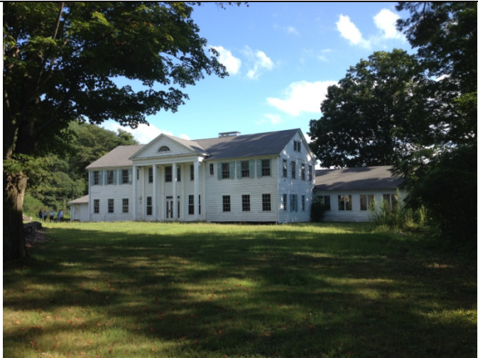
1. View from South Maple Street toward front of building
