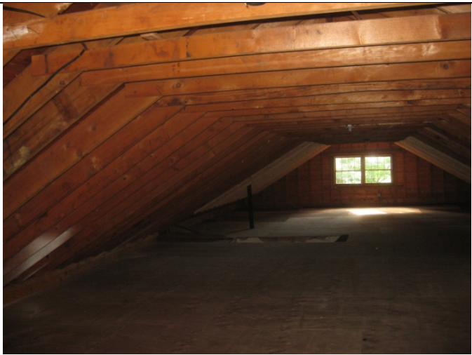
7. Attic level of main building
