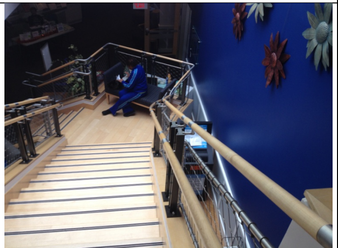
8. Stairway with sitting nook from 1 st to 2 nd floor
