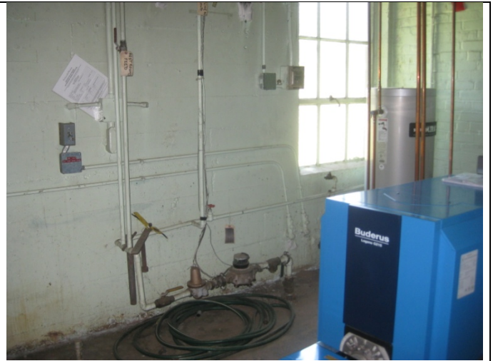
6. Mechanical room with boiler
