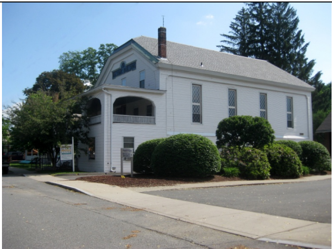
1. View from Main Street of Masonic Building
