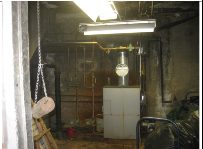
8. Existing mechanical room at basement level
