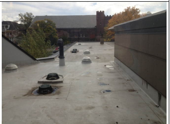
4. Roof top view with solar tubes for daylighting into the building
