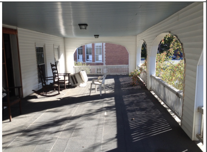
10. Porch area at second floor level
