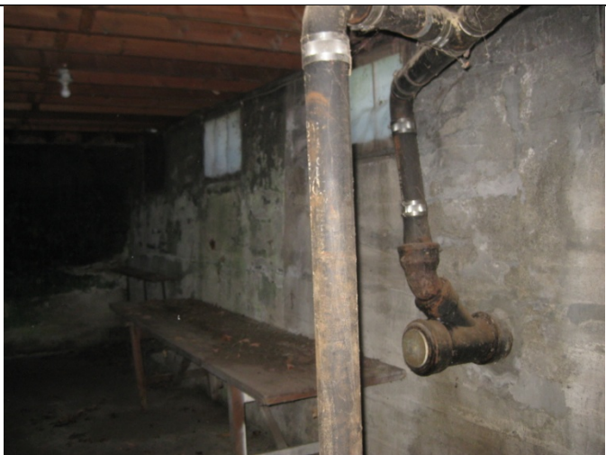
9. View of basement level
