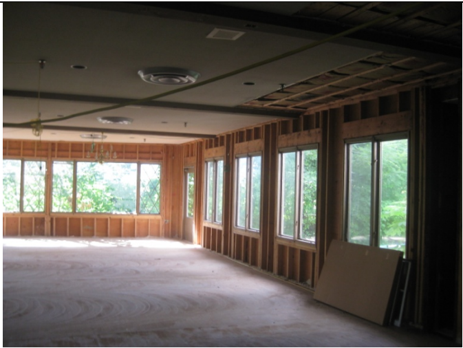
5. Former banquet hall
