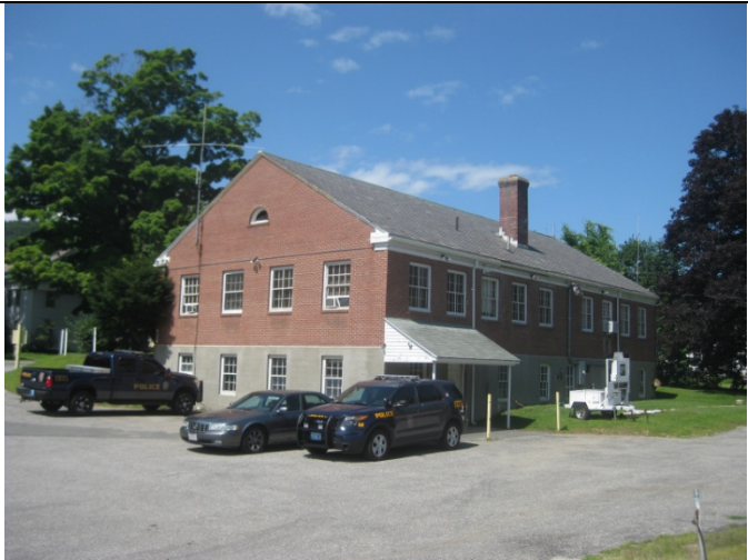
1. View from parking lot of lower level of Buckland Police Station Building
