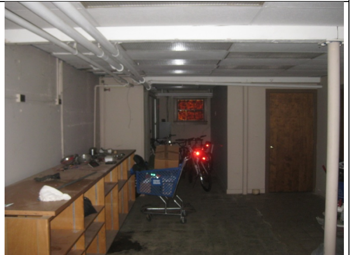
10. Main room looking toward kitchenette area
