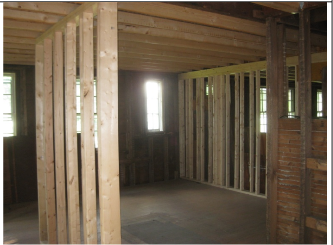
8. New walls at second floor level
