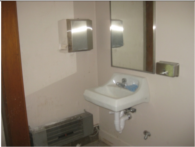
5. View of existing accessible restroom
