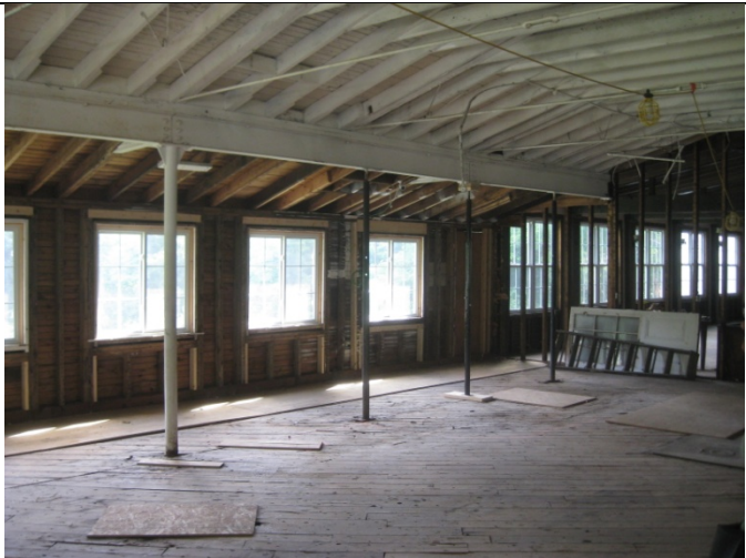
3. Former kitchen area
