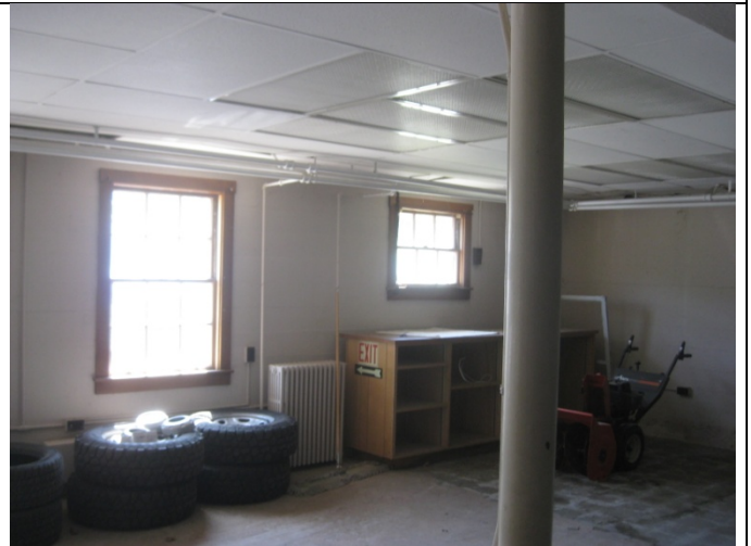
4. View looking toward south of large main room
