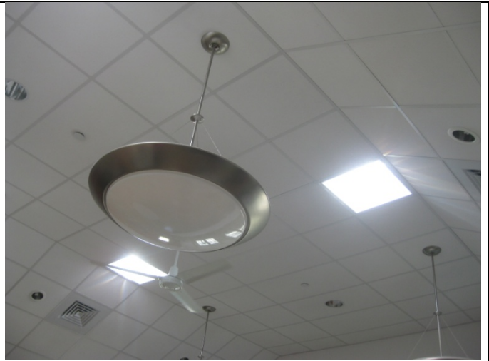
12. Interior view of light tubes providing strong natural light into building
